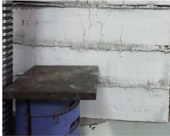
Fig.10. failure of stack bonded fiber reinforced CLC prism
